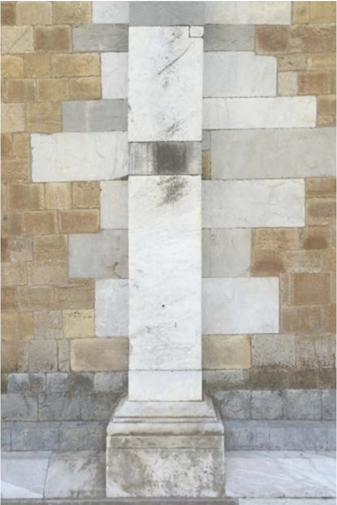
Figure 12: Reused Roman building blocks, Duomo, Pisa, Italy.
