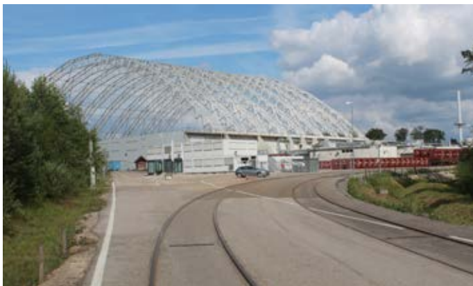
Figure 11: Cleanup and restoration of the Bonfol site, Switzerland.
