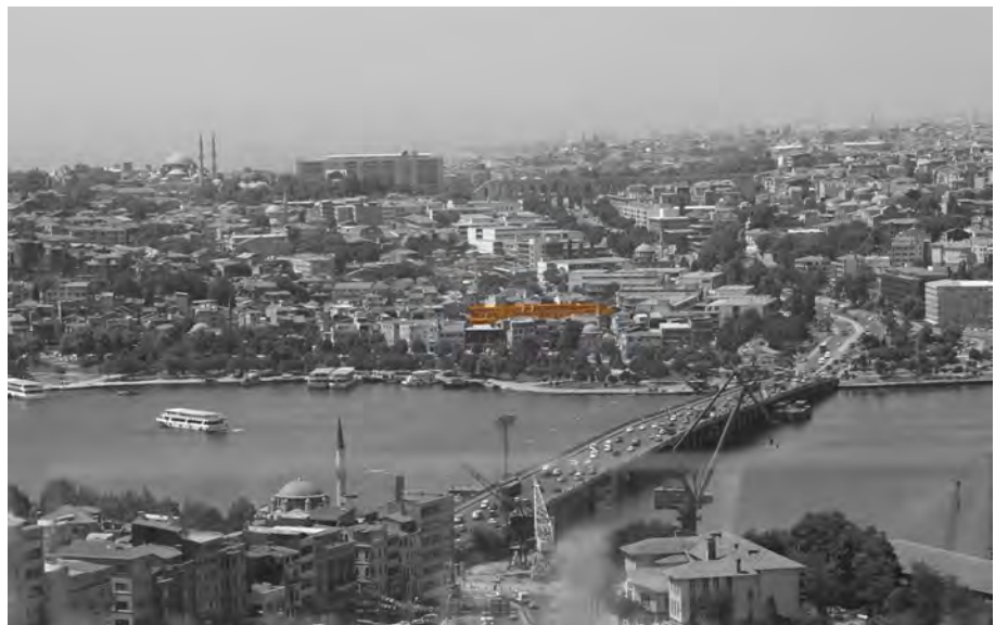
Figure 1: The Unkapanı Flour Mill in the urban context
