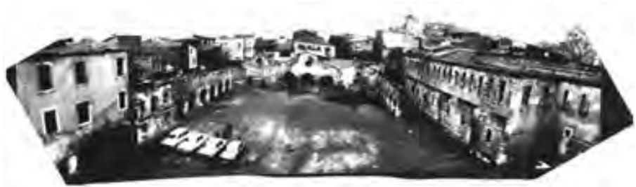
Figure 11: Unkapanı Mill's dilapidated buildings and courtyard repurposed as a parking lot, 1980, Taç Foundation Archive
